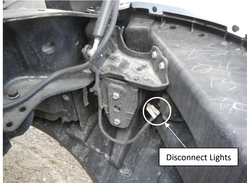
Figure 1 – Factory Driving Lights Disconnected (Passenger Side Shown).
